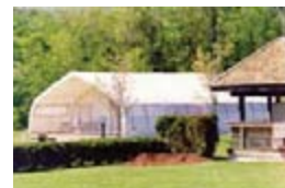
Outbuilding with an extended porch area
