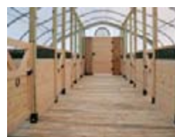
Light framed unit with stalls for livestock
